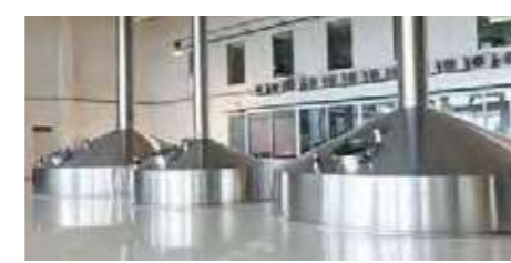
Brewery production equipment
