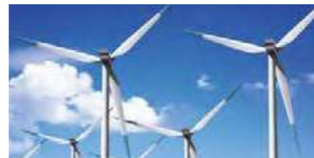
Wind turbine speed monitoring
