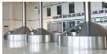
Brewery production equipment
